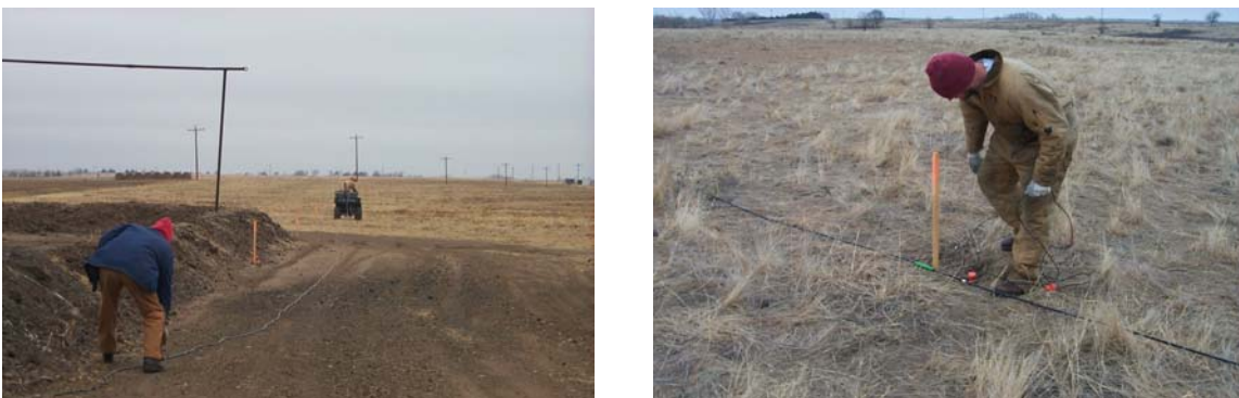
Figure 29. (left) cable laid with ATV along stakes and (right) geophones planted at surveyed stake.
