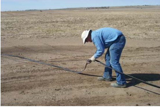
Figure 41. Installing cable protector across road.
