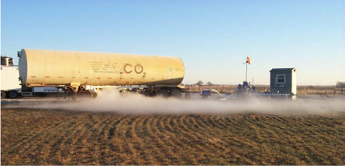
Figure 30. During normal operations CO 2 will occasionally vent from storage tanks.
