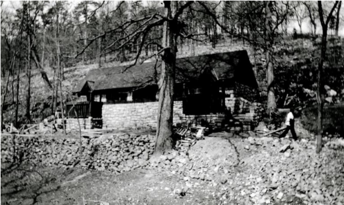
Figure 4. HS-423 after construction. A stone retaining wall and abutments were dry laid against the embankment, date unknown. View is to the north (Bishop 2015: Figure 2-60).
