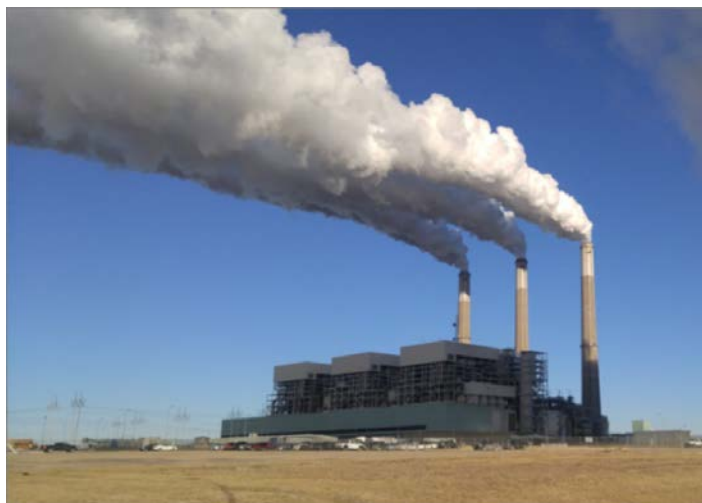
Figure 1.1. Steam billows from Westar's three 800 Mw electrical generation units on a brisk February morning at the Jeffrey Energy Center in St. Marys, Kansas. Following the kick-off meeting for ICKan., Yevhen (Eugene) Holubnyak, Petroleum Engineer, Kansas Geological Survey, Martin Dubois, Joint-PI, Improved Hydrocarbon Recovery, and Krish Krishnamurthy, head of Group R&D in the Americas for The Linde Group, visited two possible industrial sources for CO 2 , Jeffrey Energy Center and the CHS refinery in McPherson, Kansas.
