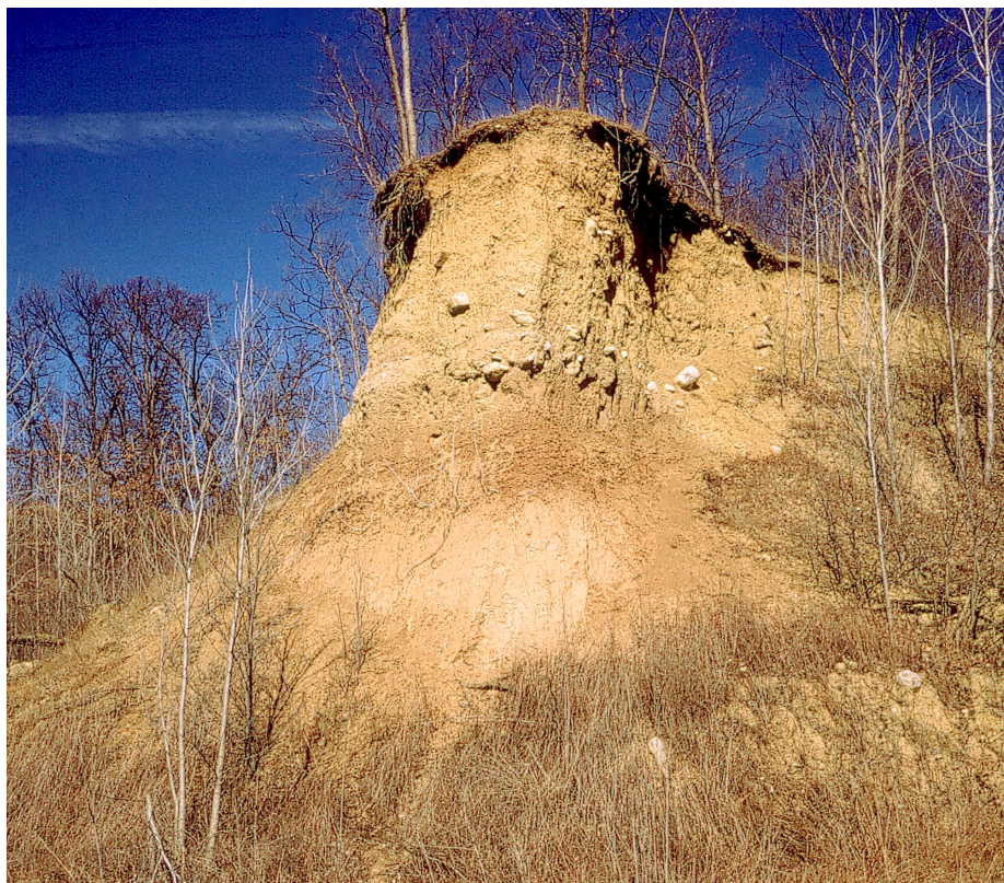
Figure 5. Because of its grain angularity and cementation, loess remains standing vertically for years in excavations and roadcuts.
